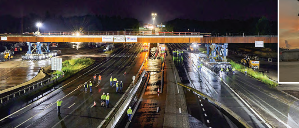
A Cometto SPMT system is used by Sarens to place a bridge section over a highway.
