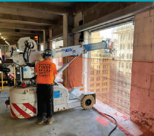
The Valla 25 is used for the installation of a Brooklyn tower's curtain wall panels.
